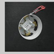
Trim the protruding part of the box, turn off the water and disassemble the flushing device.
